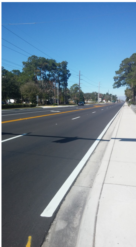
Completed construction of Wickham Road including bi-lateral turn lanes and new side-
